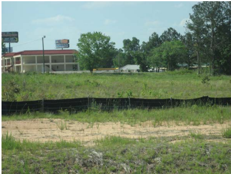
Partially cleared site
